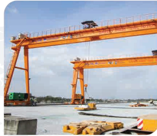
METRO LINE CONSTRUCTION GANTRY CRANE
