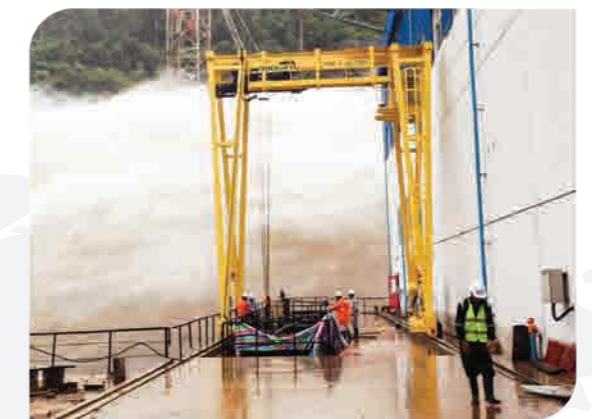
HYDRO POWER PLANT | GANTRY CRANE - Lifting capacity: 25T - Span: 9m - Lifting height: 50m
