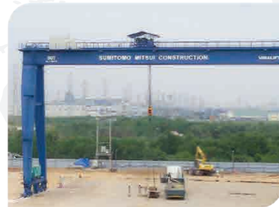
BRIDGE CONSTRUCTION | GANTRY CRANE
