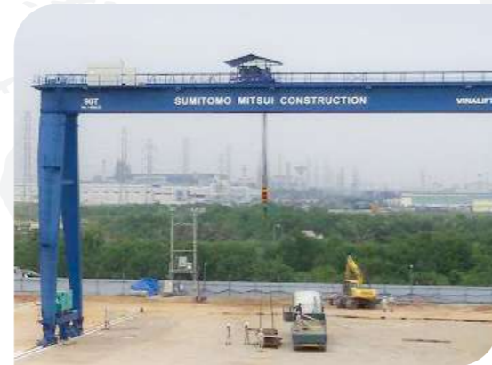
BRIDGE CONSTRUCTION | GANTRY CRANE
