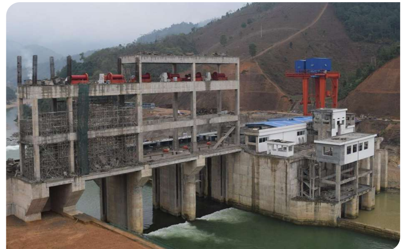
VINH HA HYDROPOWER PLANT - LIFTING CAPACITY: 2X100T/ 2X32T - SPAN: 8.5M - LIFTING HEIGHT: 40M - WORKING DUTY: 1AM
