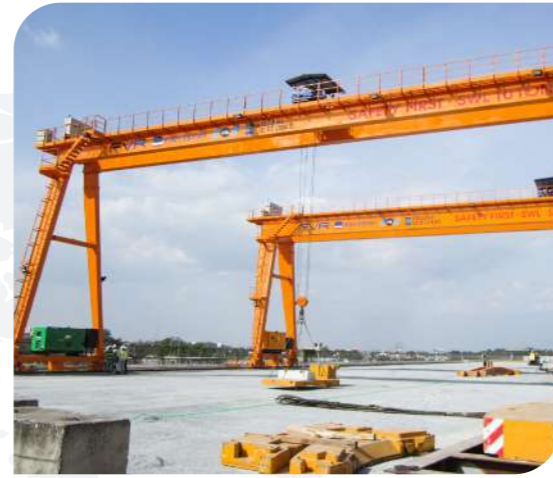
METRO LINE CONSTRUCTION GANTRY CRANE
